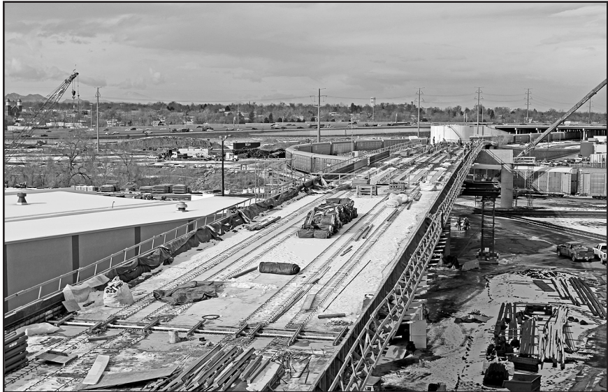
Looking northwest from near Union Station in Denver over the new bridge that will carry the RTD Arvada line above the “Buck” crossover and the BNSF shop area. – Photo © 2014 by Dave Schaaf.
